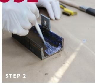
Best applied with short hard bristle brush with dabbing motion, can be applied with a short pile roller.
